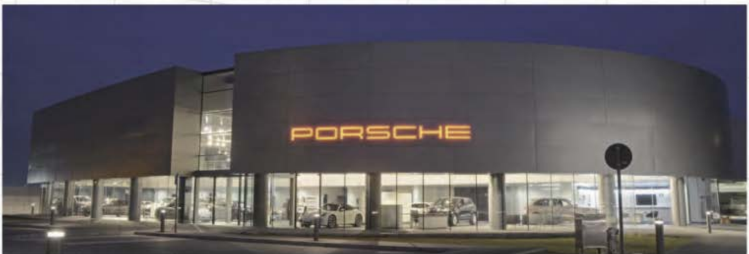
The new Porsche Showroom - Sharjah
